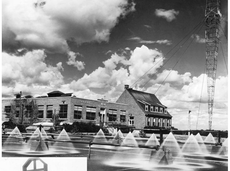
The WLW 500 kW transmitter plant, completed and in operation, 1934. The "spray pond" is part of the transmitter's cooling system.
