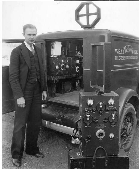
Field intensity meter and vehicle, used by WLW engineers to verify the station's signal coverage.
