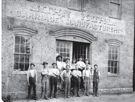
The 3-story John Kohl carriage shop was destroyed by the fire.
