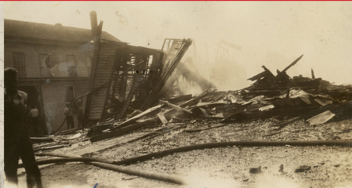
Bennett building's smoldering ruins, July 20, 1930
