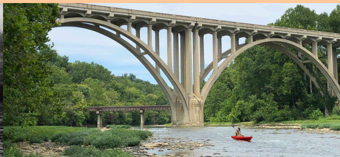
Fosters Bridge and 3-C Highway Viaduct – 2020
