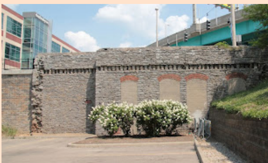
left Back side parking lot view shows the windows which allowed light to the lower level of the building. Above the bricked-in windows you can see where the floor beams attached.
